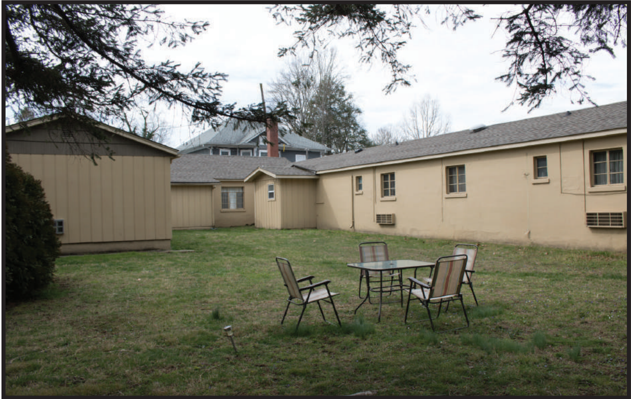
Figure 34. Circa 1960 Southeast Addition, Looking South
