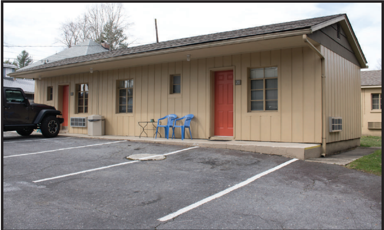
Figure 35. Circa 1960 Southeast Addition, Looking West
