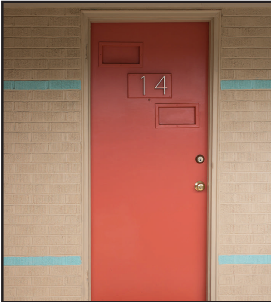
Figure 37. Room 14 Entry (in Circa 1960 Section)
