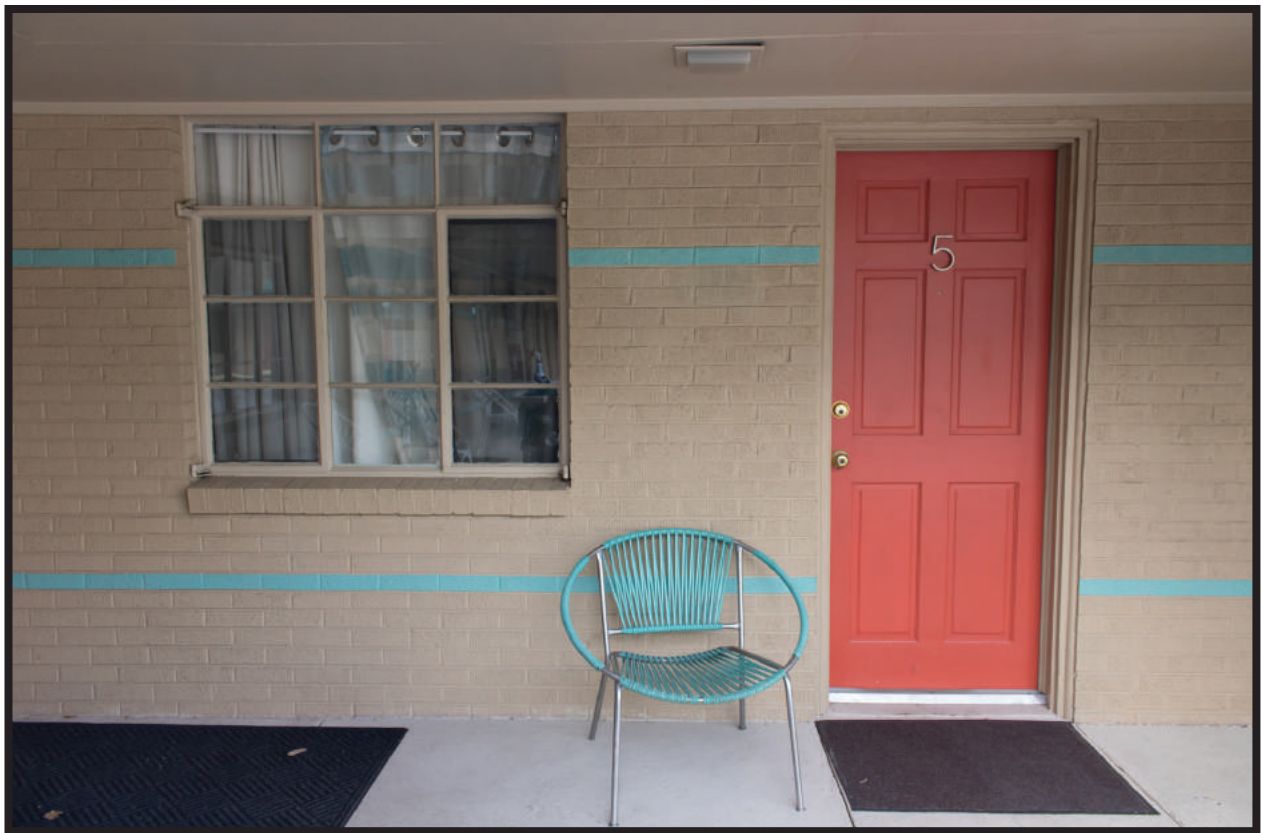
Figure 36. Circa 1960 Southeast Addition, Looking West
