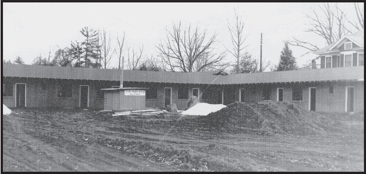
Figure 42. Sunset Motel Under Construction
