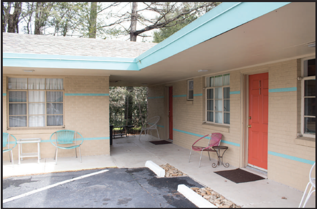
Figure 27. Breezeway at Northeast Corner Connecting 1955 and Circa 1960 Guest Rooms
