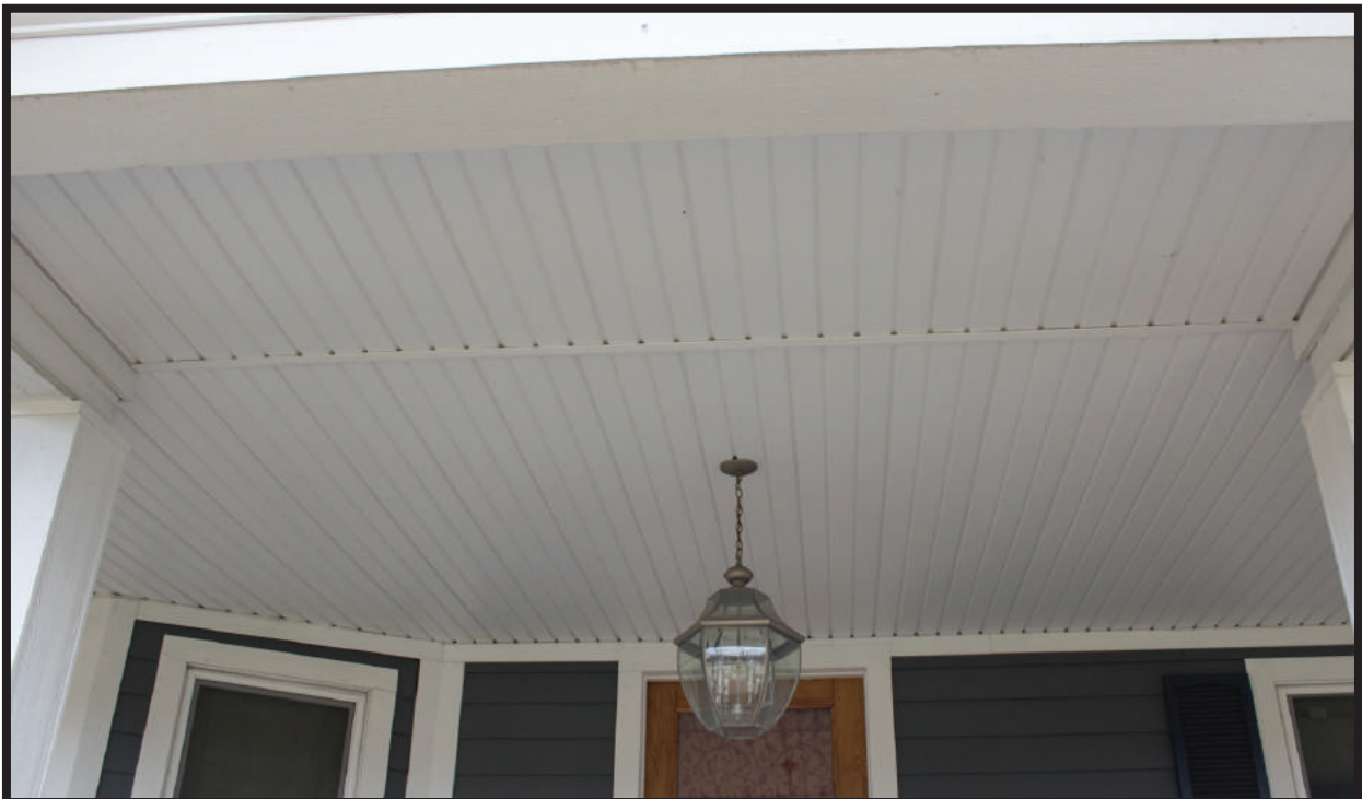
Figure 13. Detail of Porch Ceiling
