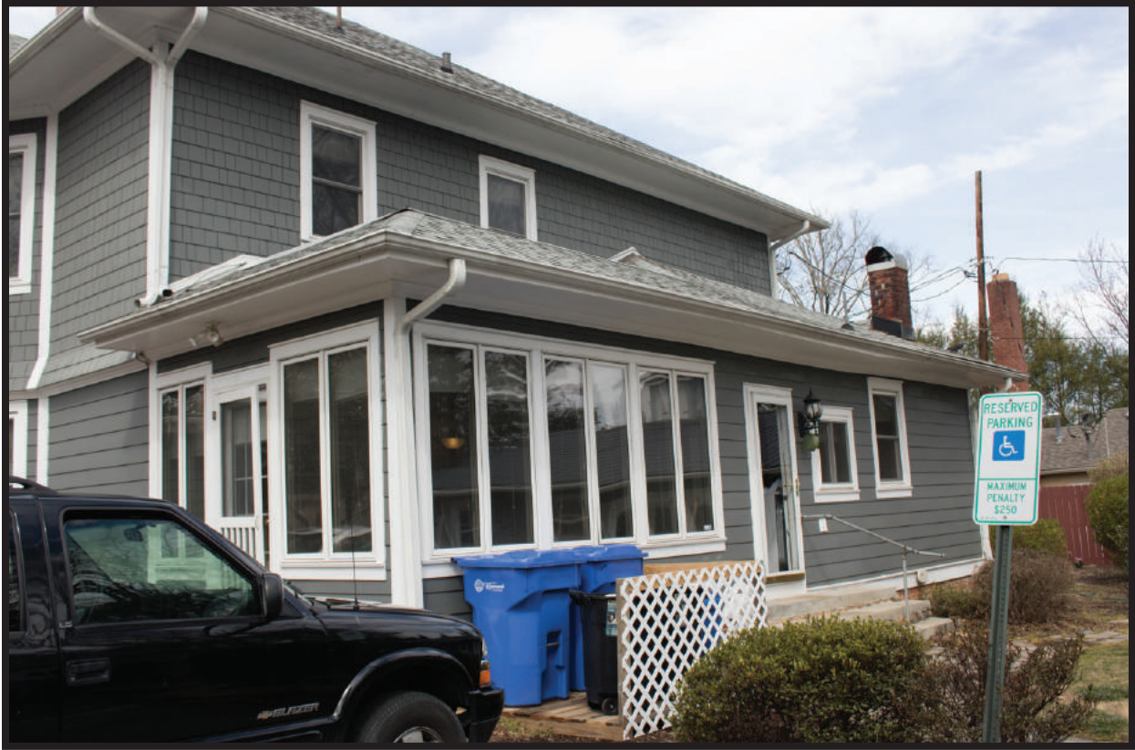
Figure 12. Rear of the House, Looking Northwest
