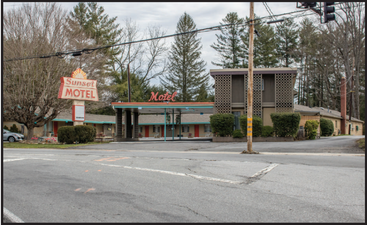
Figure 25. Front (West) Side, Looking East
