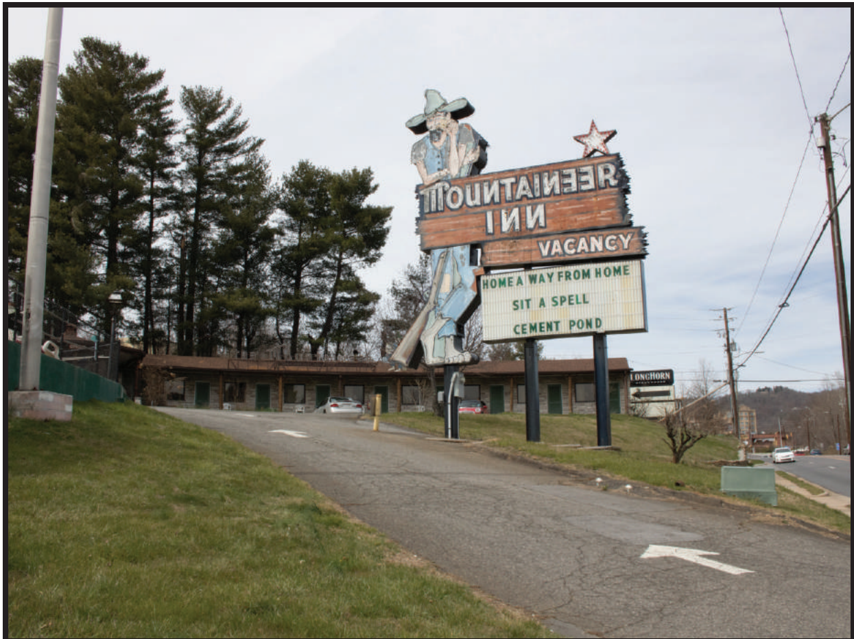
Figure 47. Mountaineer Inn, 155 Tunnel Road, Asheville, Buncombe County
